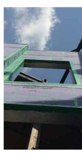
AIR-SHIELD LIQUID FLASHING is to be used as a liquid-applied flashing, compatible with the entire line of AIR-SHIELD air, vapor, and liquid moisture barriers.
