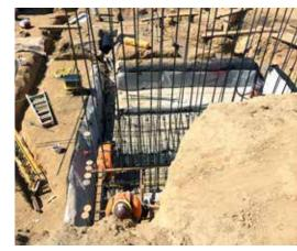
W. R. MEADOWS offers our newest addition to our complete concrete below-grade waterproofing product line with CLAY-TITE. CLAY-TITE is a dual layer waterproofing consisting of virgin HDPE (20 mil) and sodium bentonite, along with a protective layer consisting of a non-woven polypropylene.
