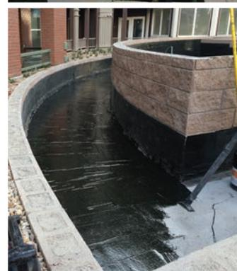
**HYDRALASTIC 836** keeps water where it belongs – whether it's applied inside, outside, horizontally or vertically! Designed with specifiers and end users in mind, this cold-applied, 98% solids, single-component compound is ideal for positive side waterproofing for foundations and in between-slab applications.
