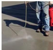
When applied to fresh concrete, SIL-CRETE helps to reduce water evaporation and improves the surface integrity of the concrete.
