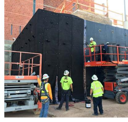
material was HRM 714, and the cold-applied material was HYDRALASTIC $_{\text{\tiny TM}}$  836.
