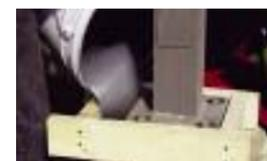
**SPEED-E-ROC™** is a very rapid hardening, very rapid setting, non-shrink, pourable anchoring cement and flowable non-shrink grout. SPEED-E-ROC will achieve 5,000 psi in one hour. SPEED-E-ROC is designed for anchoring bolts, rails, ties, threaded rods, sign posts, parking meters, street signs and ornamental steel work into concrete or other porous, structural material.
