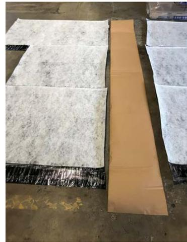
Remove the release paper on the one side of the tape and fold back to expose 6" (152.4 mm) of the rubberized asphalt and apply the PLASMATIC CORE side of the PRECON into this and roll press into place.
