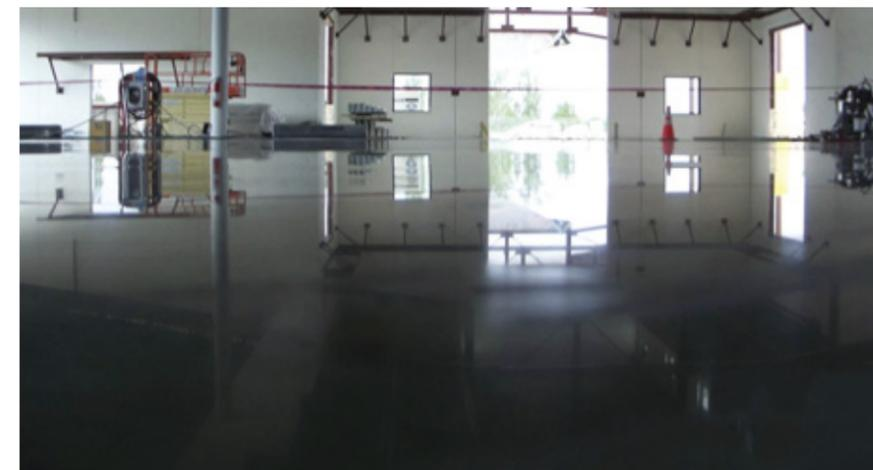
Attaining the desired level of shine in polished-concrete installations depends on the number of passes of the diamond disc grinder, as each step increasingly flattens the floor and enhances light reflectivity.
