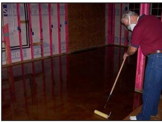
This application is part of a rebuilding of a home destroyed by Hurricane Ike. The first photo shows the neutralization of the acid stain with water. The others show the application of DECRA-SEAL.
